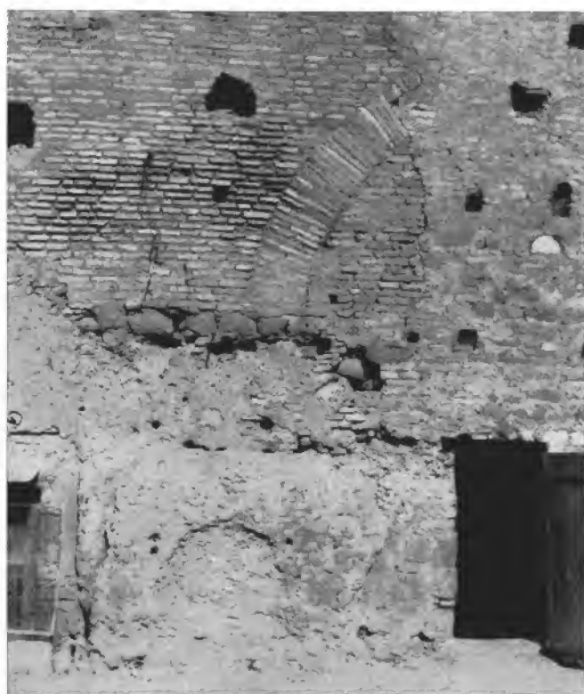
Fig. 239. S. Prisca, Part of south wall with relieving arch
